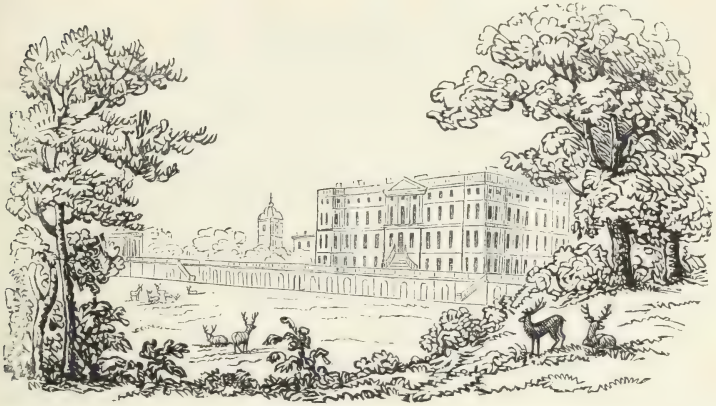
[Fig. 84. View of Burley, with the low brick terrace walls removed, and a stone terrace wall substituted.]
